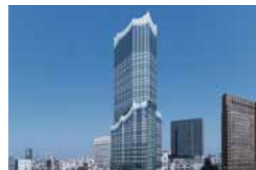
©TOKYU KABUKICHO TOWER
